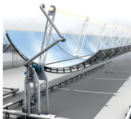
With the parabolic trough power plant, collectors concentrate solar energy onto a receiver tube positioned in the focal line and heat up the oil flowing in it. For high efficiency, all troughs have to be continuously adjusted to follow the sun's path and be focused exactly on the receiver tubes. This is achieved by magnetically coded position and angle measurement systems BML that are positioned directly on the rotating shaft.
